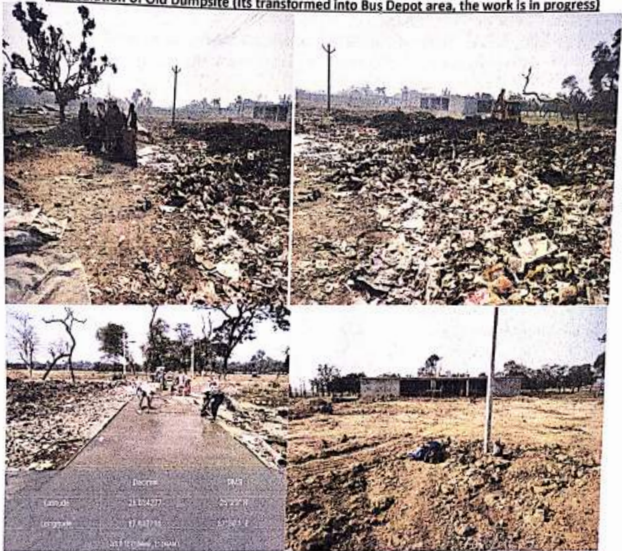
Remediation of Old Dumpsite (Its transformed into Bus Depot area, the work is in progress)
